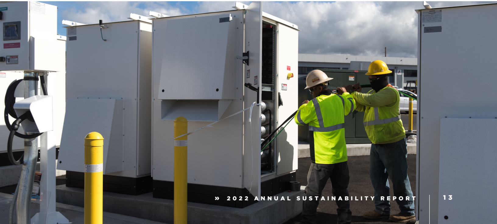
Workers construct new electric bus chargers at the Department of Transportation's Kalihi-Pālama facility. Credit: Office of Climate Change, Sustainability, and Resiliency
