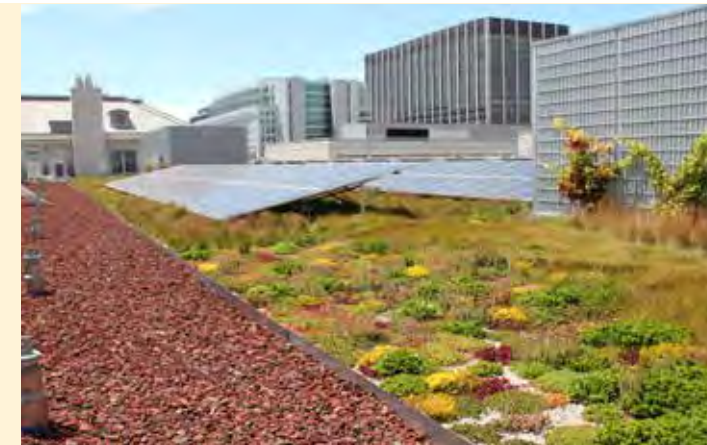
A living roof atop the U.S. Federal Building at 50 U.N. Plaza in San Francisco, CA.
