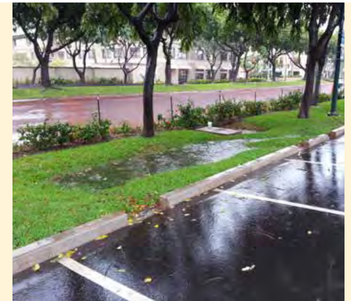
Rainfall runoff at the Kapolei Police Station directed off the parking lot into a landscaped area that is designed to hold, filter, and infiltrate the stormwater better managing water quality.
