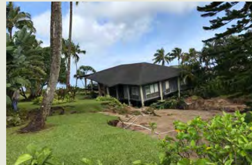
A collapsed house near the beach at Hanalei Bay, Kaua’i
